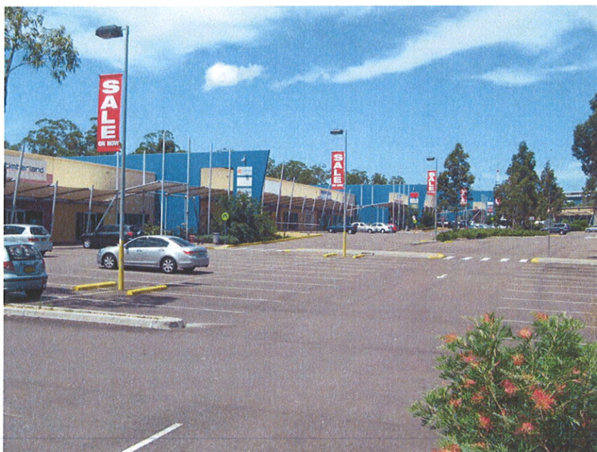
Figure 7 – View of Retail/ Bulky Goods Warehouse development to the north of the Site
